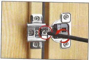
Depth adjustment by eccentric cam: + 2.5 mm (+ 3/32) / - 0.5 mm (- 1/64")
